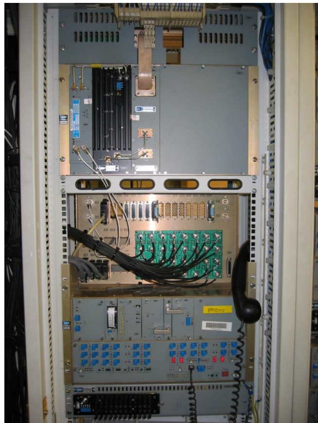
Figure 1: Siae 7.5GHz 16 x 2Mbps digital microwave radio system - all indoor solution (late 1980s)
