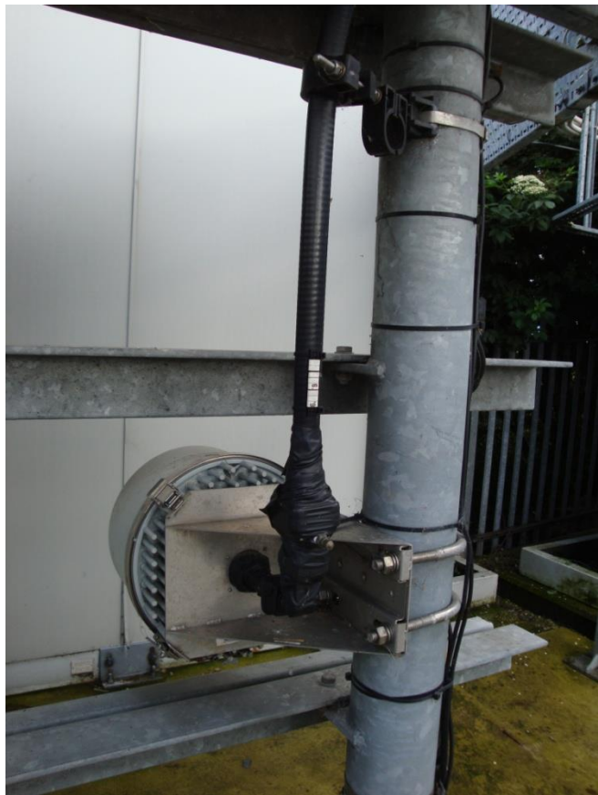
Figure 3: PCOM ODU, 13GHz ODU - split mount systems (IDU/ODU), with waveguide between ODU and antenna (mid 1990s)
