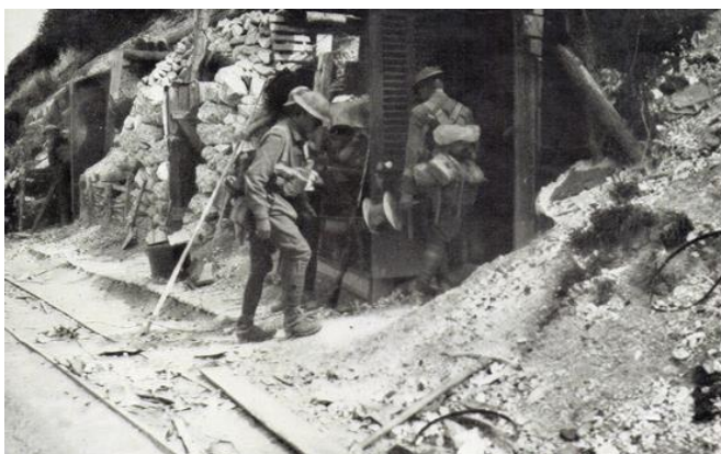
Figure 2: Laying telephone cables in the trenches
