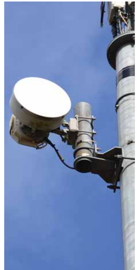
Figure 3: Direct mount arrangement with ODU connected to parabolic antenna
